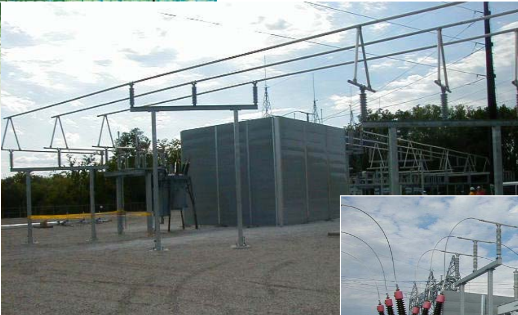
SL Barrier Panel, 20' (High) 30' x 30' L-Shape Kentucky Utilities, Louisville, KY Results: 17dBA reduction at property line, overall 13dB at 125Hz
