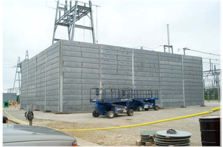
SL-R Barrier Panel, 26' (High) 60' x 75' L-Shape Commonwealth Edison, Casey Road, Chicago, IL Results: 19dBA at property line, overall 13dB at 125Hz
