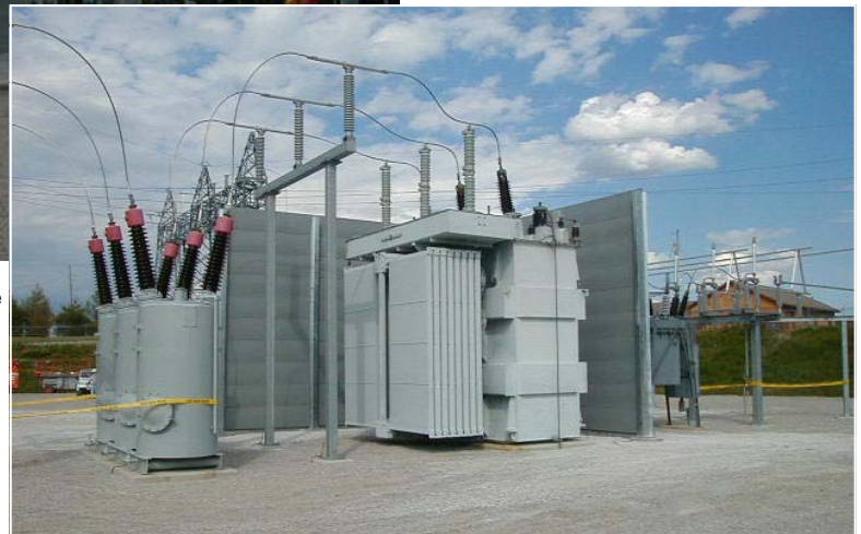
SL Barrier Panel, 20' (High) 30' x 30' L-Shape Kentucky Utilities, Louisville, KY Results: 17dBA reduction at property line, overall 13dB at 125Hz
