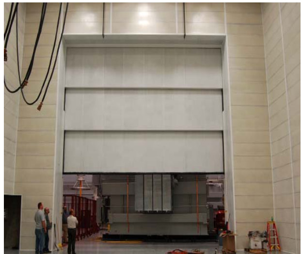
Sectioned Door, STC 5130' x 34' high, NIC 47. Telescoping Vertical Lift Door installed in Noise Barriers' 63 Hz cutoff 20' x 60' 45' high Hemi-Anechoic Chamber.
